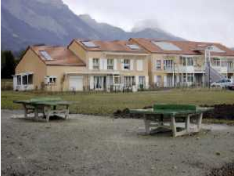
OPALE SOCIAL HOUSING : ENERGY CONSUMPTION FOLLOW-UP
