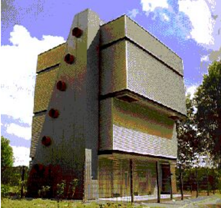
KWK-ANLAGE IN ARNHEM
